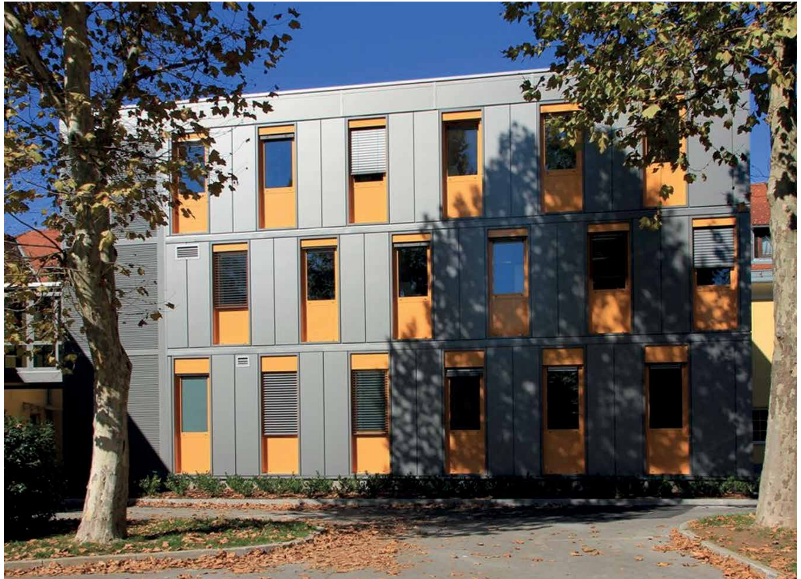
Construction featuring 21 Trimo MSS modular units, 2010
